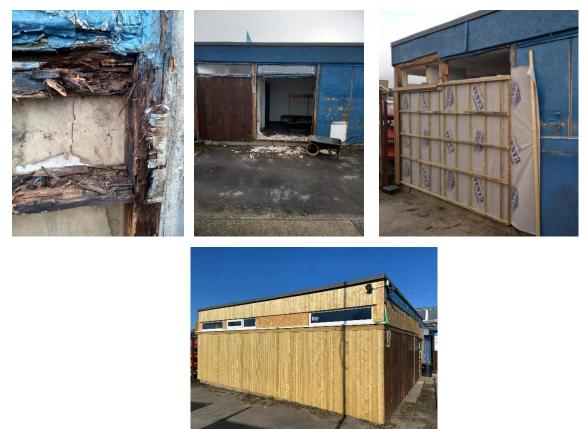
Tony Dufton is in the process of rectifying this replacing p[plywood cladding with treated timber and new upvc windows This will prevent any further deterioration and also looks a great deal better.
